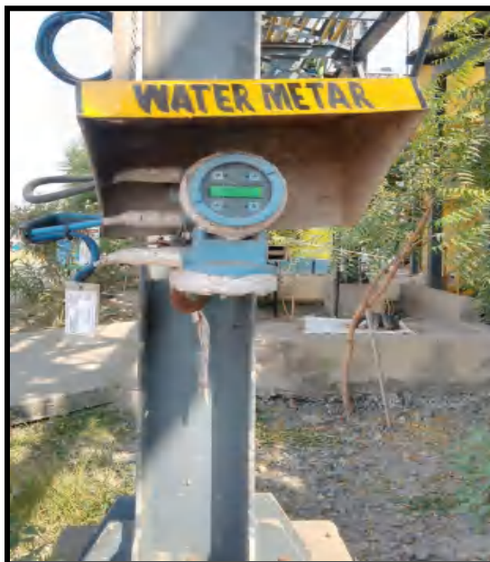
Flow Meter at RO Inlet (CT Blowdown)
