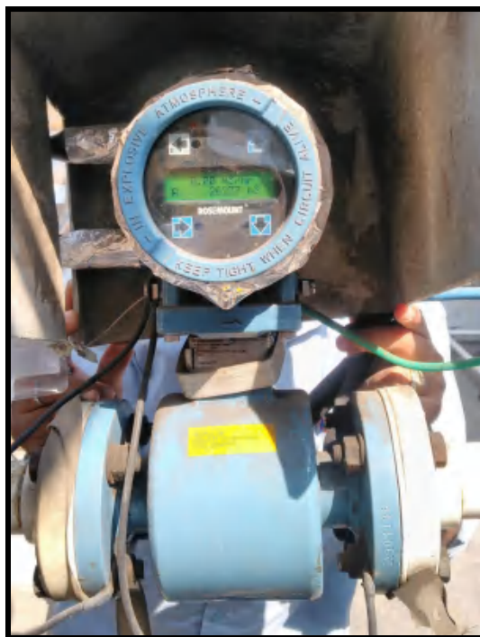
Flow Meter at RO Outlet
