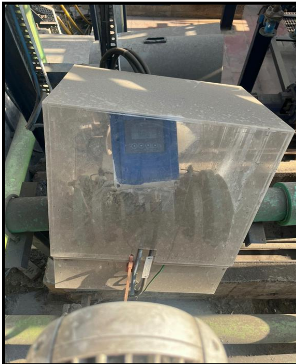
Flowmeter at NCT Discharge Point
