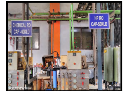
RO Process (Chemical)-60 KLD & HP RO-50KLD
