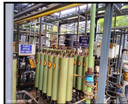
Utility RO-1 - 150 KLD & Utility RO-2 - 550KLD
