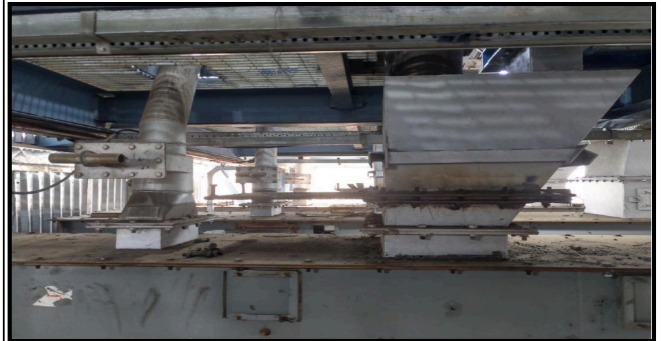
Automated Lime feeding system for controlling SOx emission.
