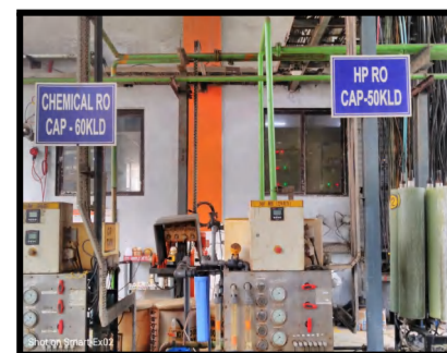
RO Process (Chemical)-60 KLD & HP RO-50KLD
