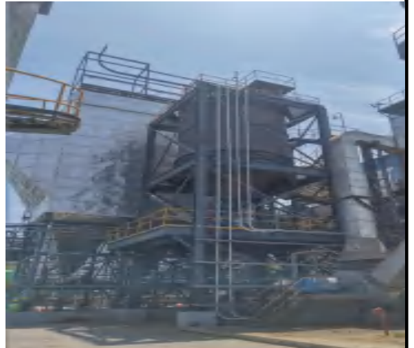
Silo installed for fly ash storage and dusting free truck loading
